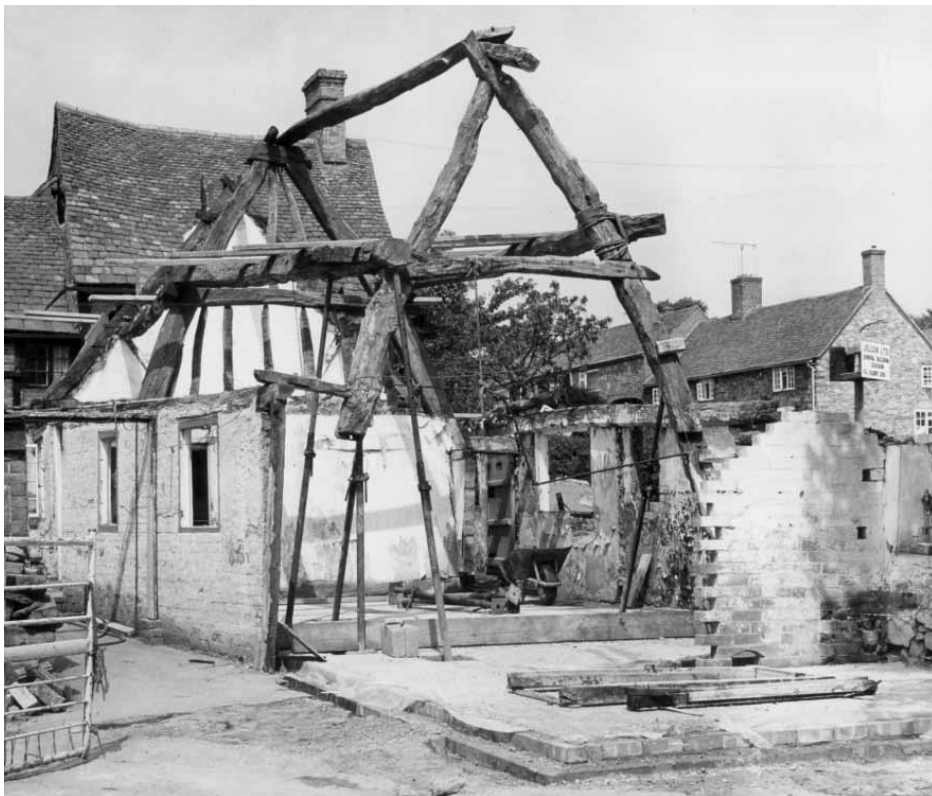
Remnants of cruck frames revealed during the re-building of the Dairy Farm, 28 Main Street, in 1975.
