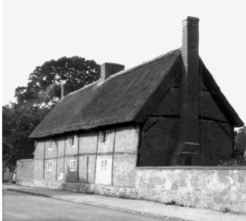
Workhouse Row (now demolished) shows well the box frame timbers in this picture.
