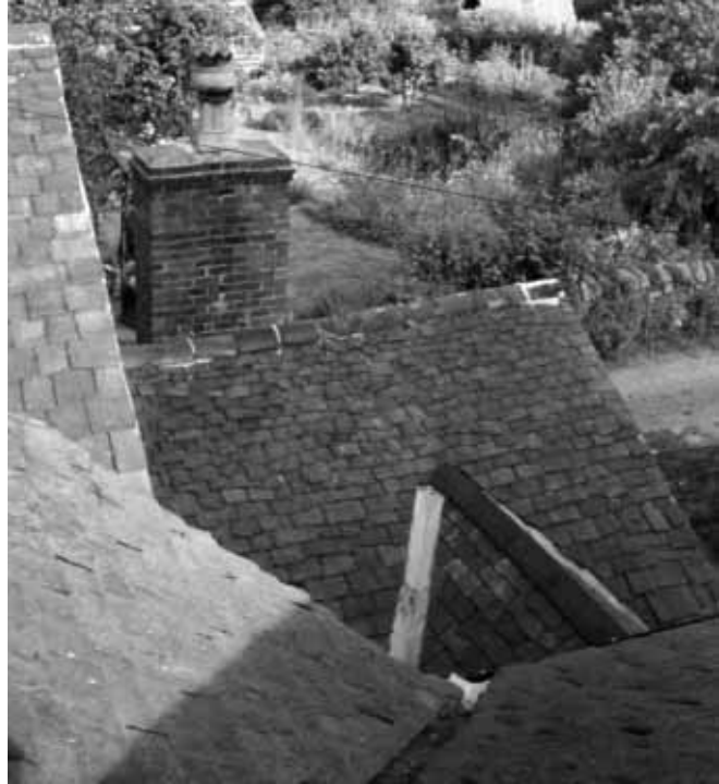
Above: Swithland Slate roofs at Beech Farm.
