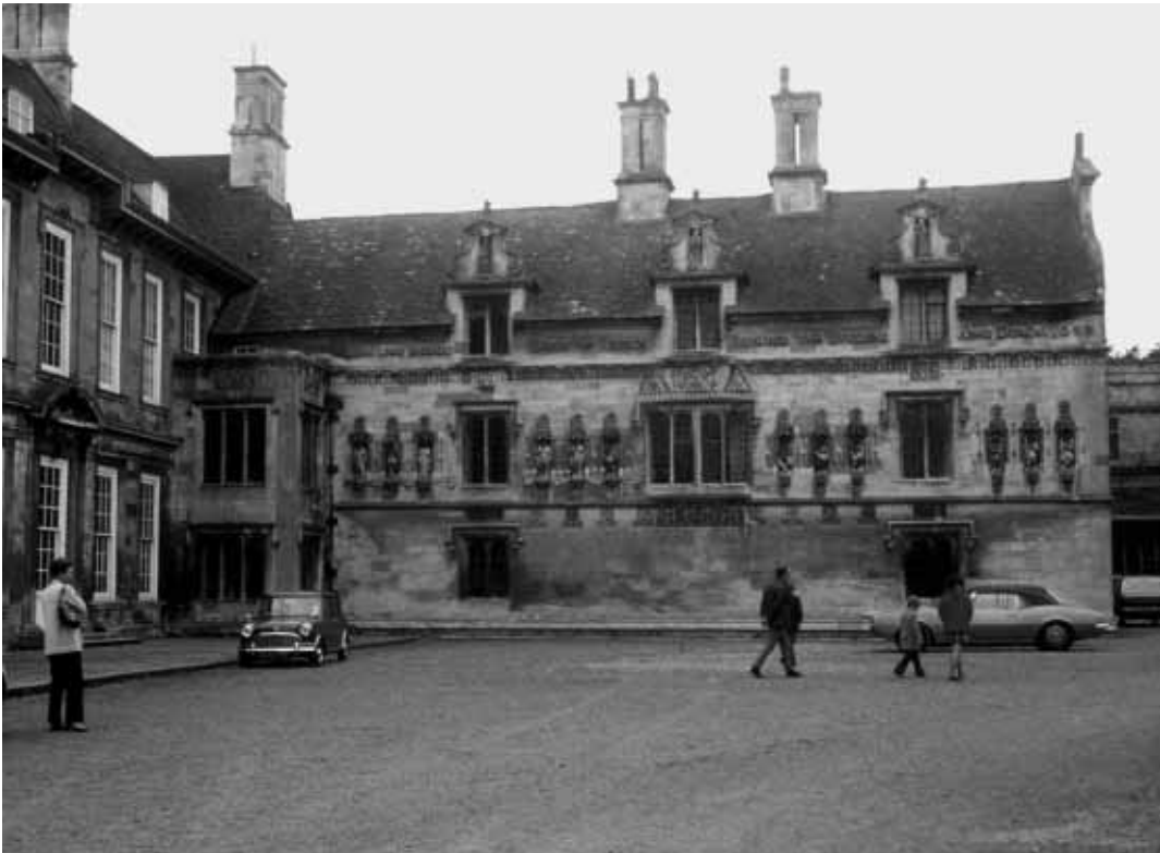
6. The east wing of Stapleford Park, known as Lady Abigail's Wing, dates originally from 1500 and was reconstructed in 1633. Between the windows on the first floor are twelve niches containing statues, the six to the right dating from about 1500 and the six to the left from 1633.
