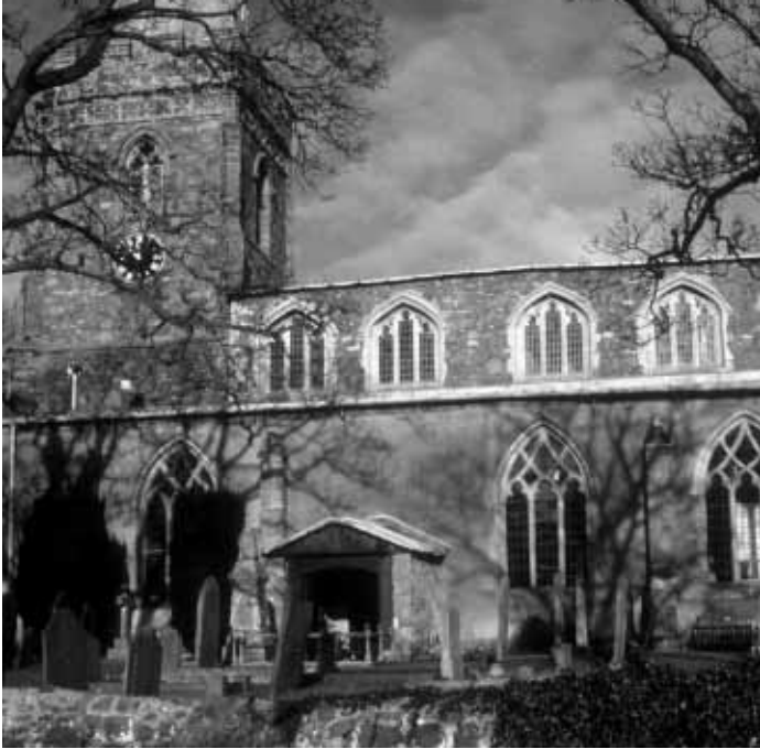
Figure 36 (right): The Perpendicular clerestory of St Mary, Queniborough, Leicestershire rises above the nave and its windows flood the nave with light.
