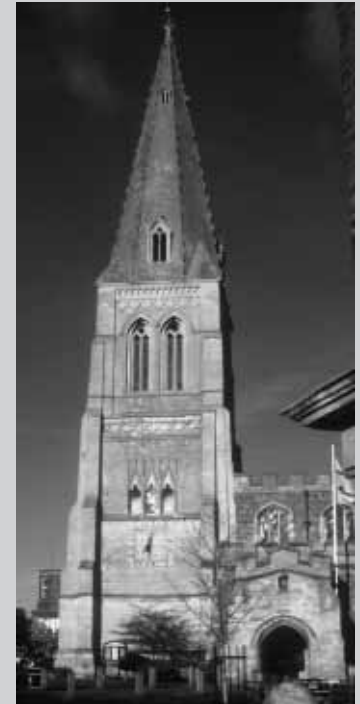
Figure 17 (top left): A typical broach spire rising from the tower by means of half pyramids of masonry, St Mary, Barkby, Leicestershire .
