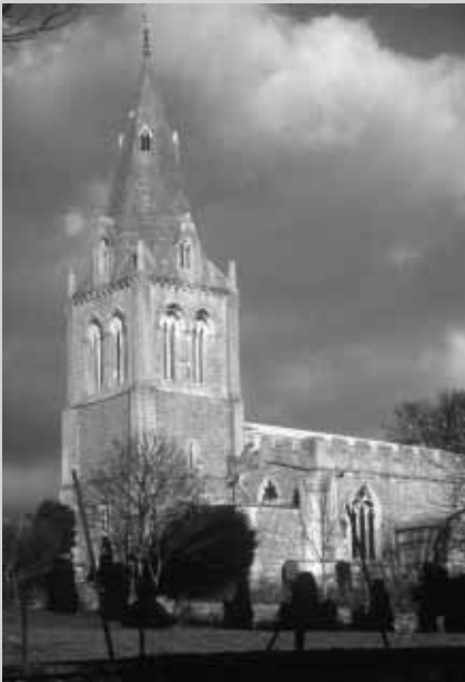
Figure 17 (top left): A typical broach spire rising from the tower by means of half pyramids of masonry, St Mary, Barkby, Leicestershire .
